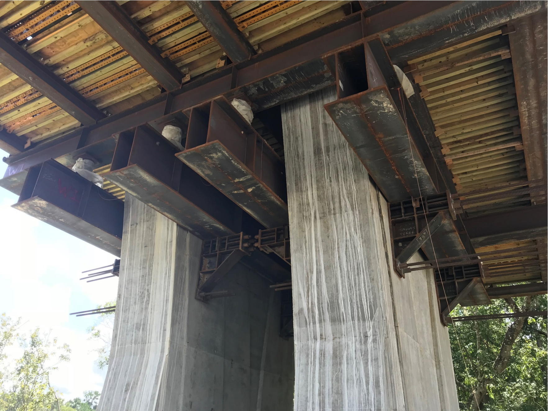
Photo courtesy of Superior Construction.
