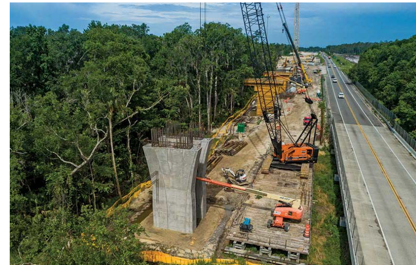
Photo courtesy of Superior Construction.
