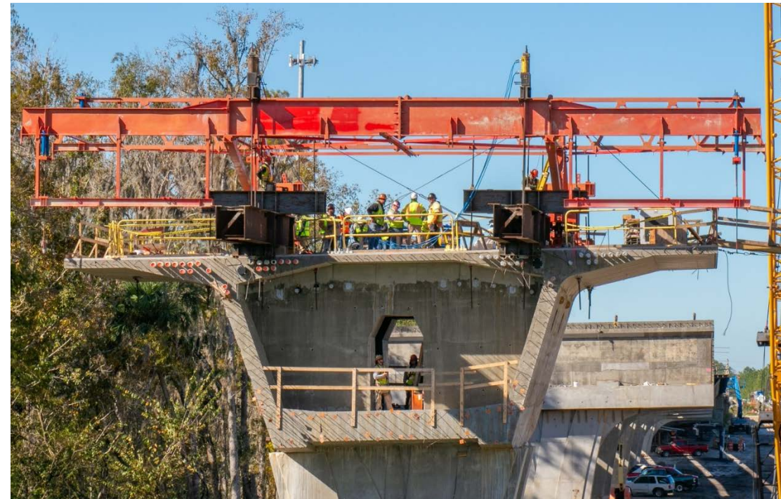
Photo courtesy of Superior Construction.
