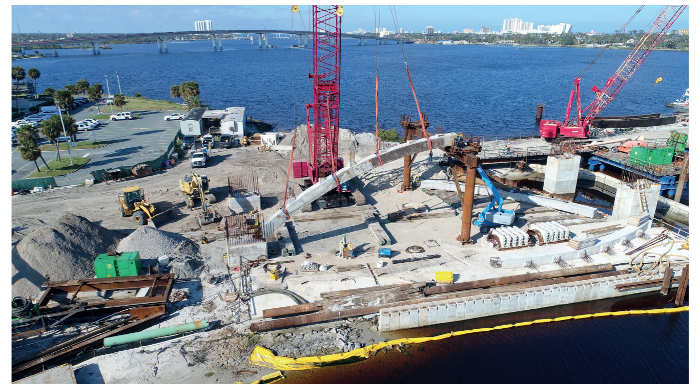
Fig. 15 Construction Site Photo of the Erection of First Precast Arch Rib [1]
