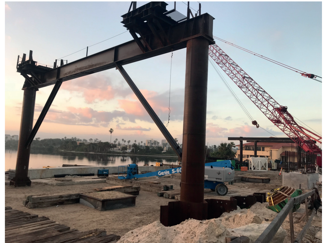
Fig. 14 Approach Span Falsework Tower
