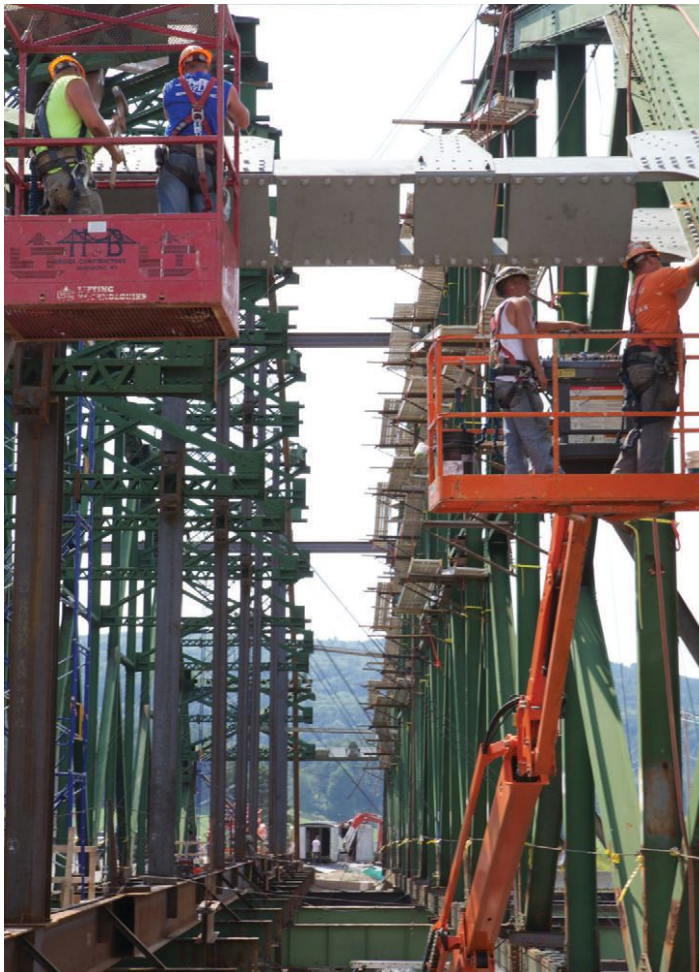
▼ Erecting the new steel. Approximately 120 tons were added.
