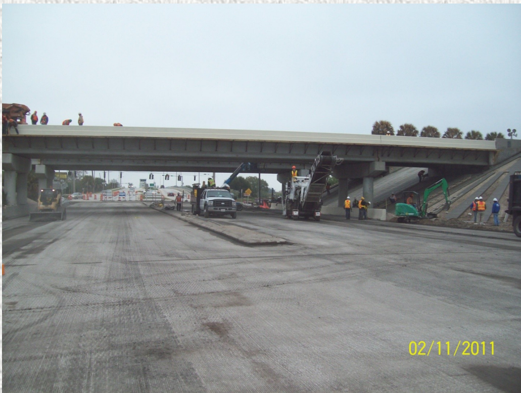
Milling of SR 3 was completed the next day.
