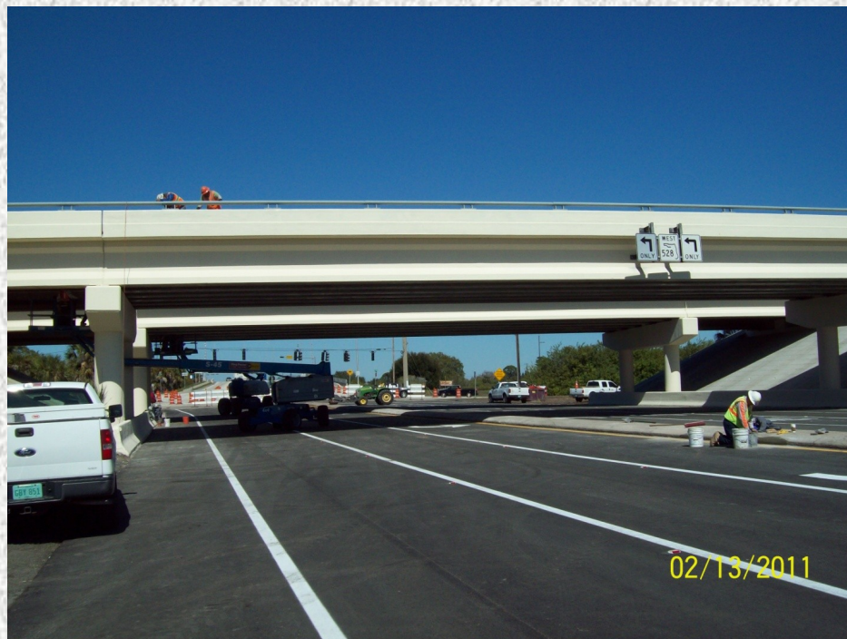
The completed bridges.
