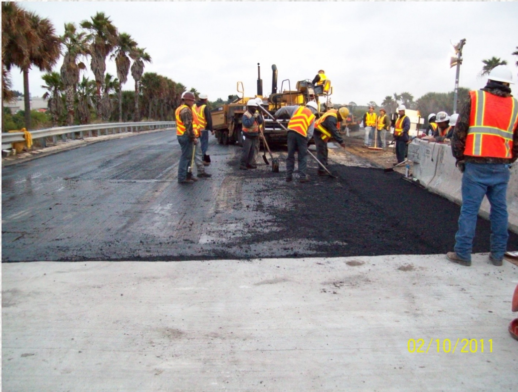
Once the milling was completed, paving of SR 528 began.
