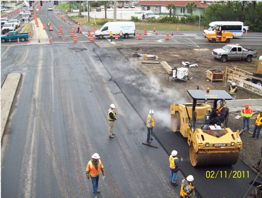
Once milled, SR 3 was paved.
