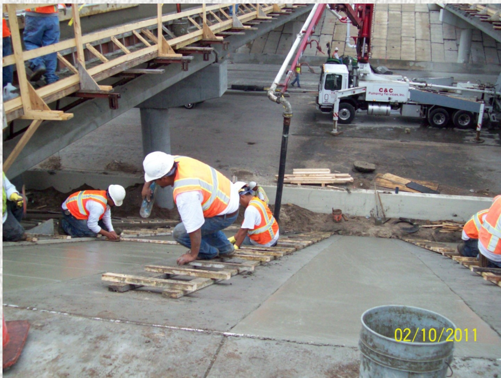
The concrete slopes were also being placed.
