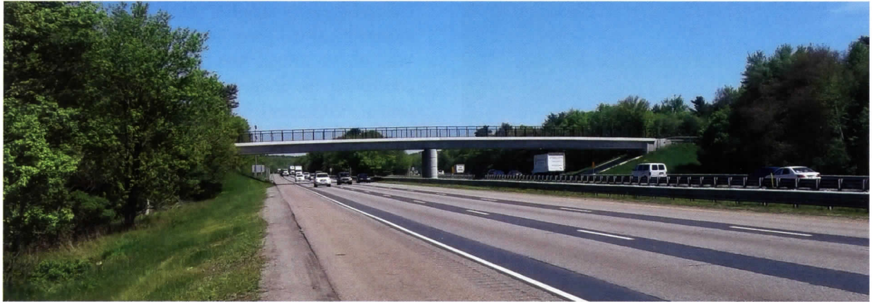
The new precast concrete channel bridge (bottom photo) and the original steel I-girder bridge (top photo) and are shown for comparison. The new channel bridge provides nearly 2 ft of additional clearance over the original bridge without increasing the roadway profile on the bridge.
