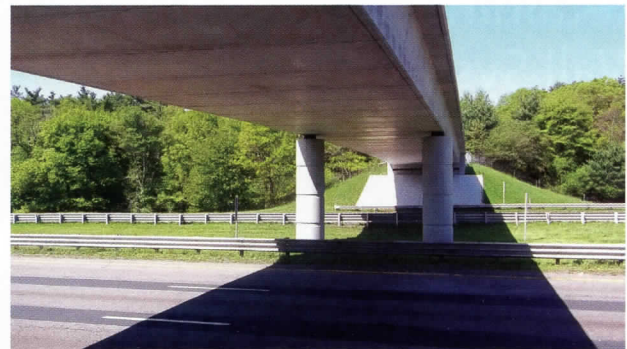
Underside view of completed bridge.
