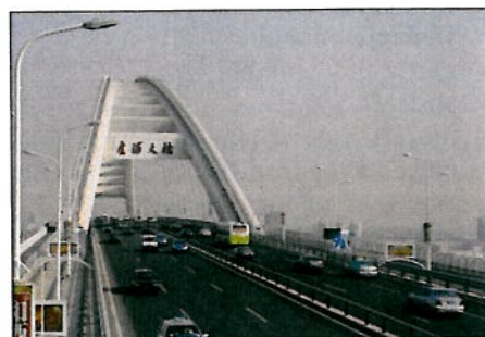
The Lupu Bridge
