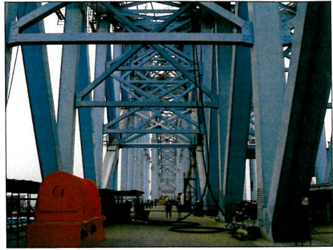
Dashengguang Bridge under construction
