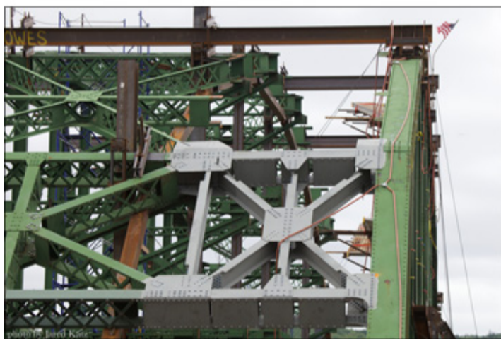
Photos: Credit Jared Katz: Top-view from east 12' separation; bottom-new brace
