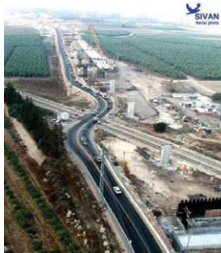
Benyamina Bridge, Israel. Photo courtesy of SIVAN
