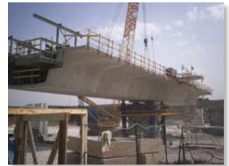
Temporary support for Cantilever Construction Section 18, Israel.
