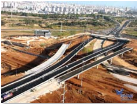
Completed Road 431, Israel. Photo courtesy of SIVAN.
