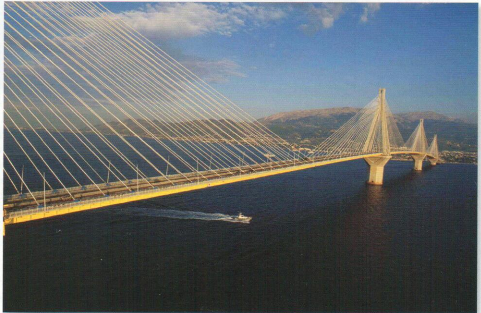
The Rion-Antirion Bridge in Greece, officially the Charilaos Trikoupis Bridge, is the longest multi-span cable-stayed bridge in the world. It is the result of close interaction between concept and construction methods.
