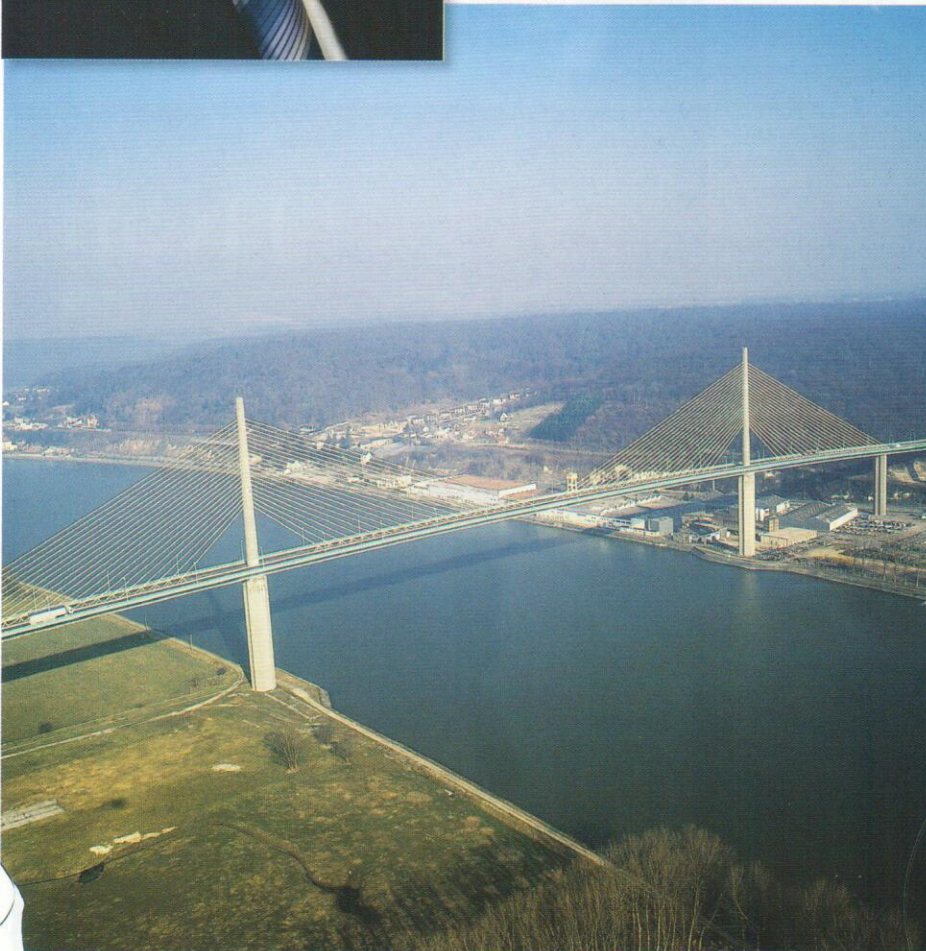
The Brotonne Bridge in France, completed in 1977, is the world's oldest cable-stayed bridge with concrete aprons. Jacques Combault calls it "the father of the Sunshine Skyway Bridge."
