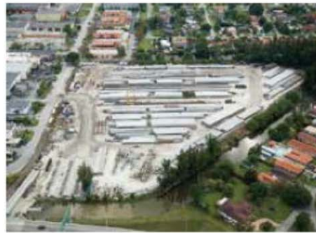
17-acre casting yard for Florida-I Beams, Prestressed Concrete Piles and MSE Wall Panels, located within the project limits. Photo courtesy of Smith Aerial Photos.
