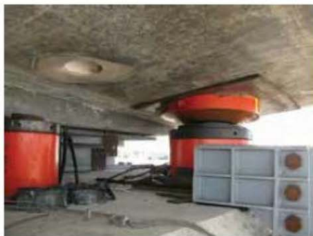
Pier cap/temporary erection jacks
