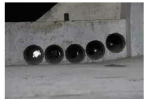
The diabolos eliminated the need for schedule 40 pipe, reduced the segment weight, allowed for variable tendon geometry and continuous external tension ducts.
