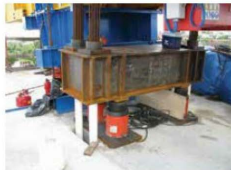
Temporary vertical tie down system.
