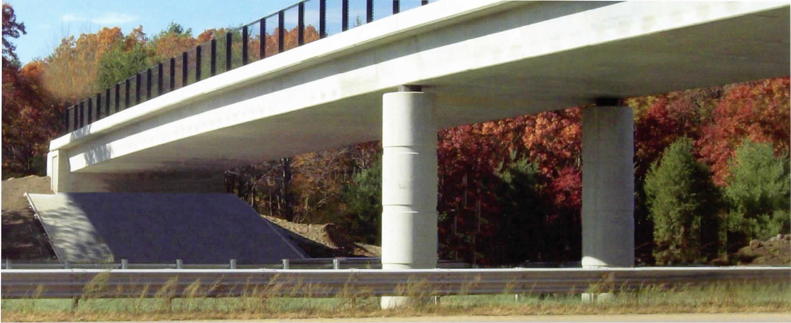
Photo courtesy of MassDOT (Massachusetts Department of Transportation.)
