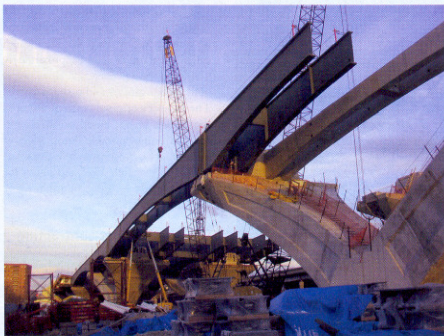
Steel plate girder superstructure placed on v-shaped piers.
