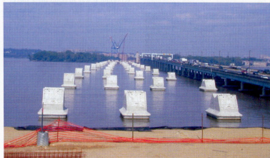
Completed foundations and pedestals from the Maryland approach.
