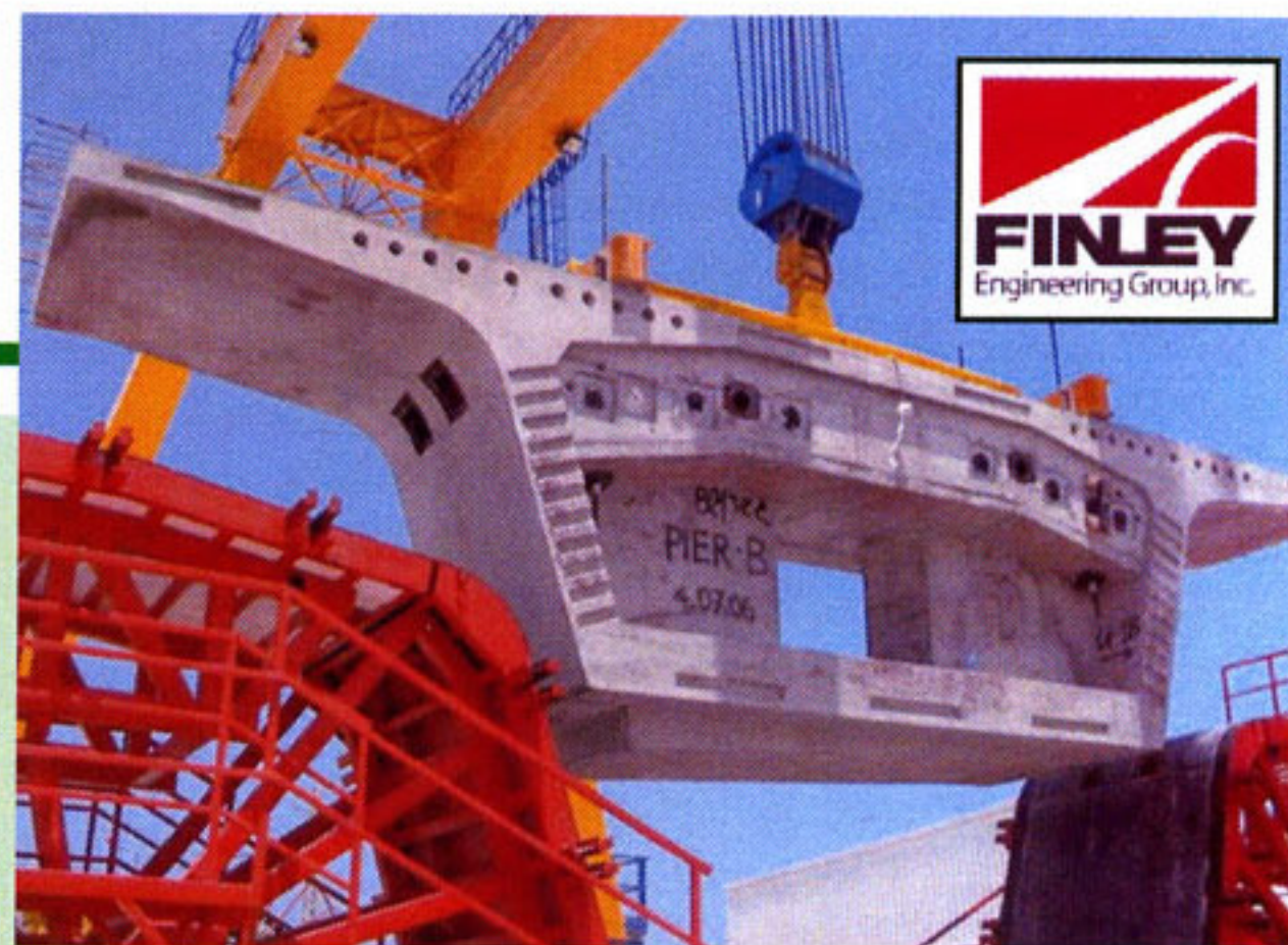
Precast pier segment for an interchange bridge on Israel's Road 431 project
