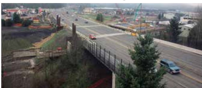
The deck is ready for casting concrete.
