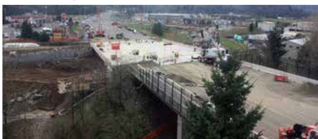
The new bridge is in its final location.
