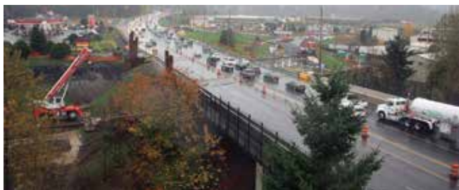
Construction of widened substructure begins on the left side.
