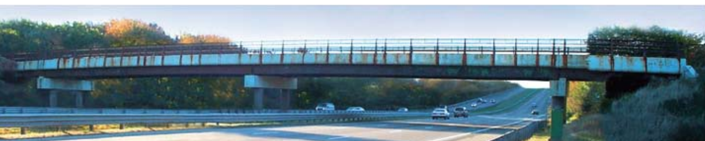
Figure 5 - Existing Bridge. (Illustration courtesy of International Bridge Technologies, Inc.).
