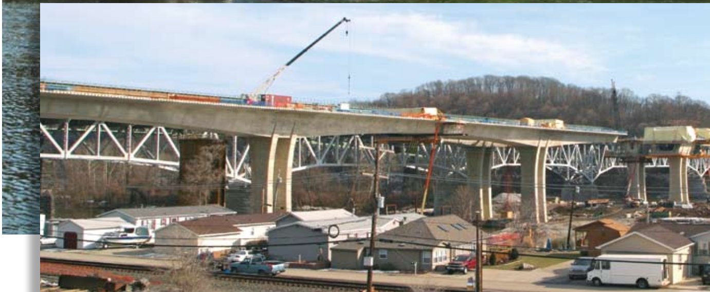
Figure 11 - (Photo inset) July 2009 - Concrete segmental cantilever construction proceeds out from the piers, nearly 100' above the Allegheny River. A stone texture on the piers will be stained to complement the surrounding landscape. (Photo courtesy of FIGG).
