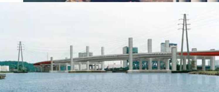
Figures 8 and 9 - The Pearl Harbor Memorial Bridge shown in these renderings will be a 10-lane, 1,013' extradosed structure. Construction is expected to begin in December 2009. (Illustrations courtesy of URS Corporation).
