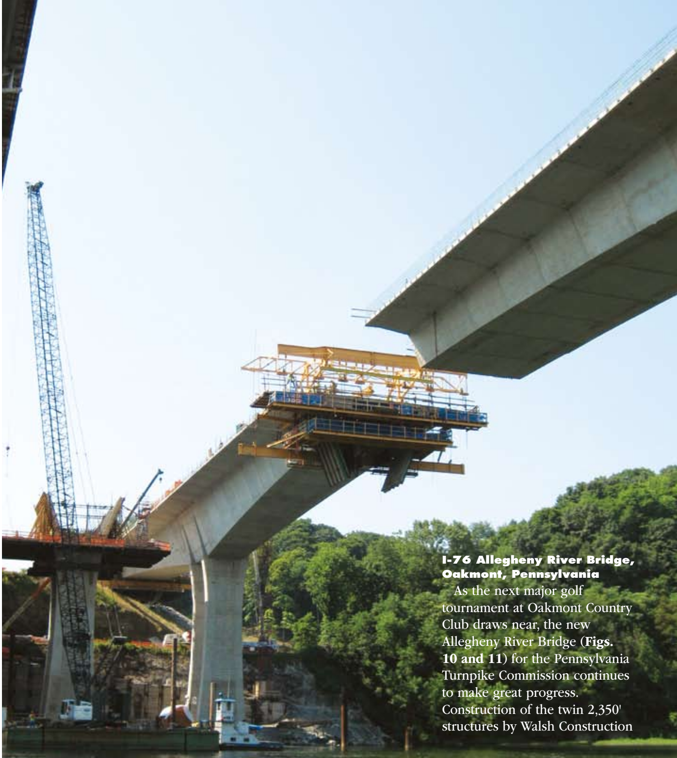
Figure 10 - (Photo top) February 2009 - Long, open variable depth spans are built using concrete segmental balanced cantilever construction to maintain mobility and preserve the environment. (Photo courtesy of FIGG).
