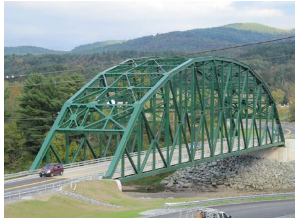
Completed bridge. This was the first time the side-launch technique has been tried on such a large bridge.
